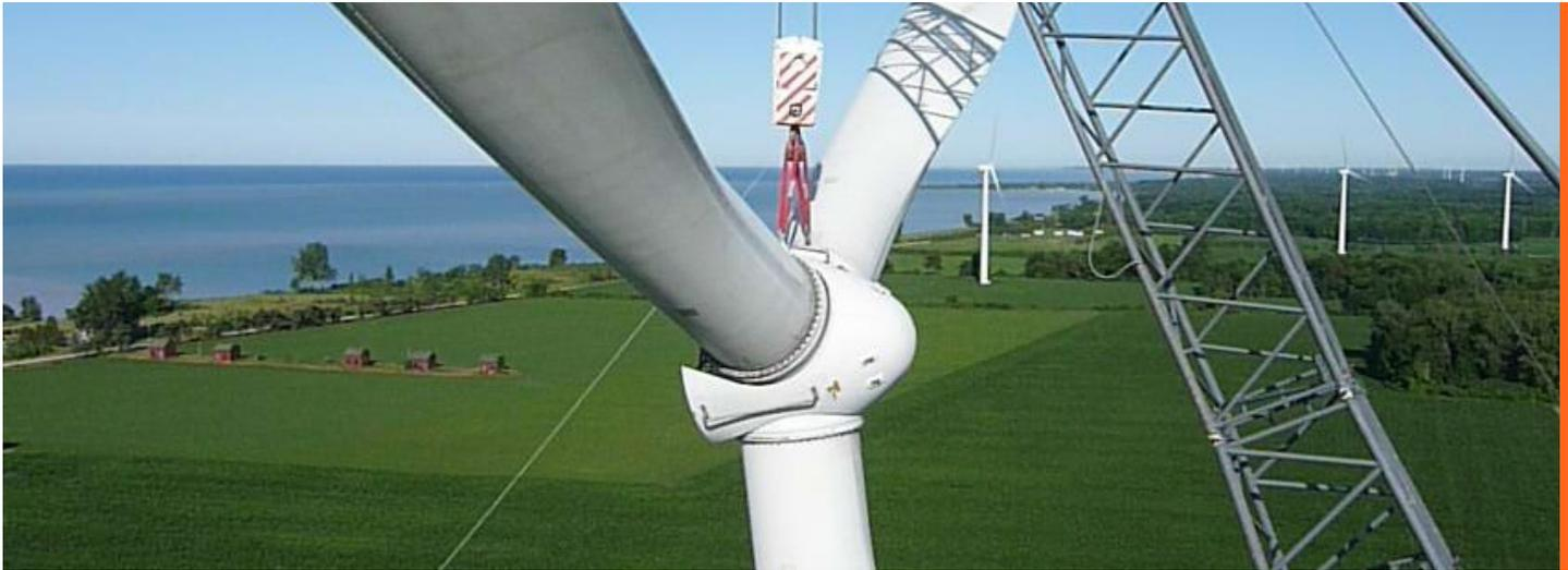
All together, the three phases of the Buffalo Atlee wind farm are located on 7 quarter sections, and will include 10 to 14 total turbines, approximately 100 to 120 m in height from the ground to the nacelle (the “hub height”), where the blades connect to the tower. The blades will each be approximately 65 to 75 metres in length, and each tower will have a generating capacity of around 3.5 to 4.5 MW.
